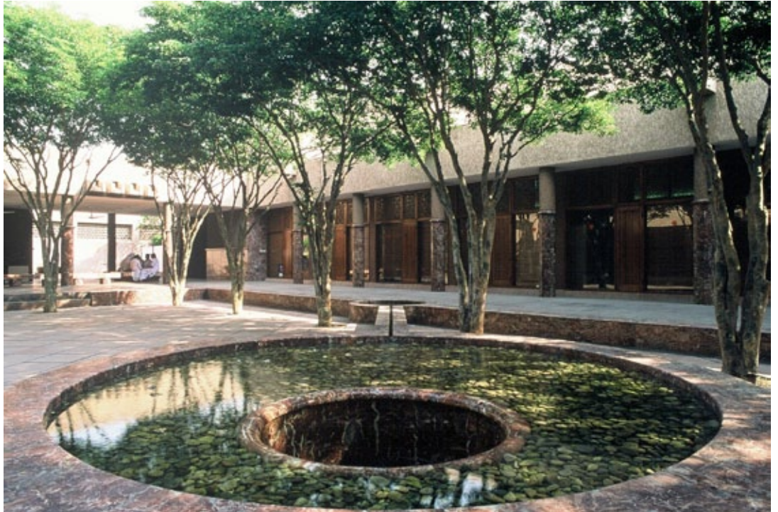
At the Aga Khan University in Pakistan, we designed water features in strategically placed courtyards to passively cool the local environment in an area where air conditioning was not feasible.
