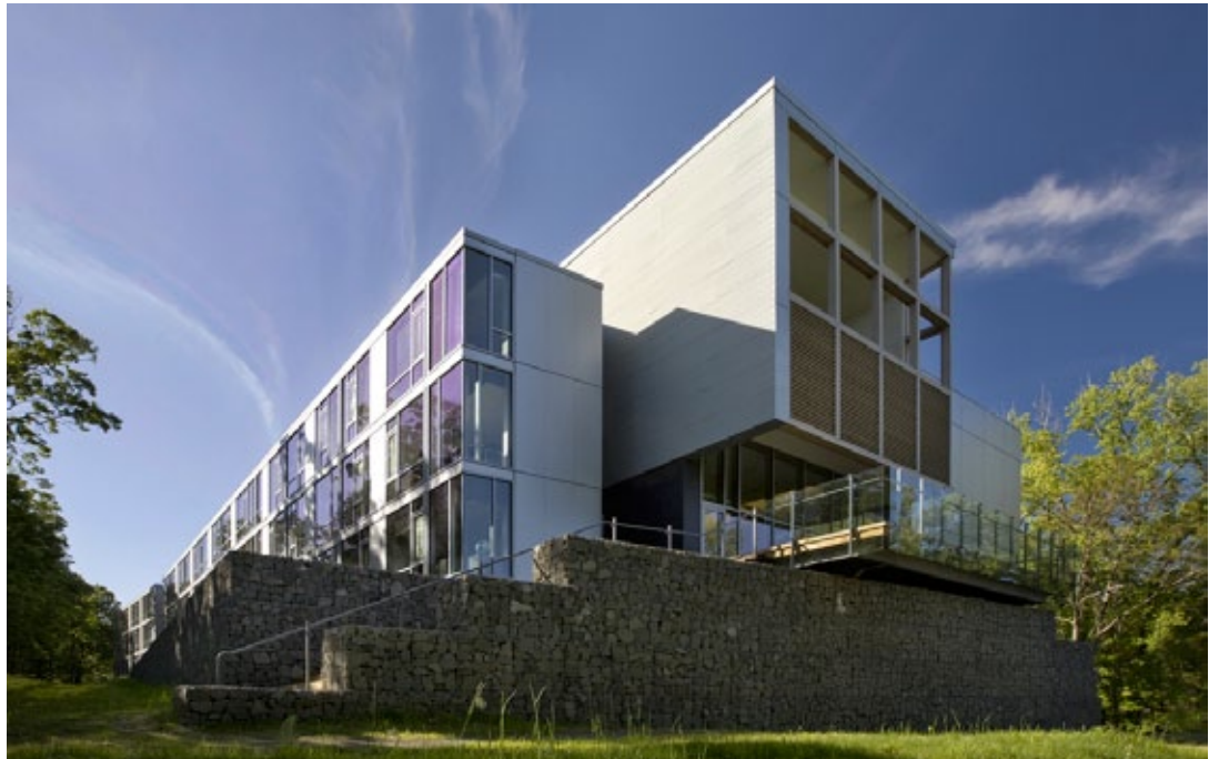
Columbia University, Gary C. Comer Geochemistry Building at the Lamont-Doherty Earth Observatory, Winner of the Boston Society of Architects, AIA/New York and EPA Award for Sustainable Design in 2009 and a Merit Award for Excellence in Sustainable Design and Development from IDID in 2010. LEED Silver Certified.
