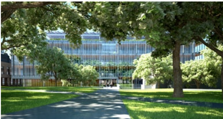
Duke University, Environment Hall, The Nicholas School of the Environment: One of the primary goals was to express the School's pedagogical mission by employing sustainable building systems that optimize energy use and water conservation while serving as a teaching tool for the school and its community. Pursuing LEED Platinum Certification.
