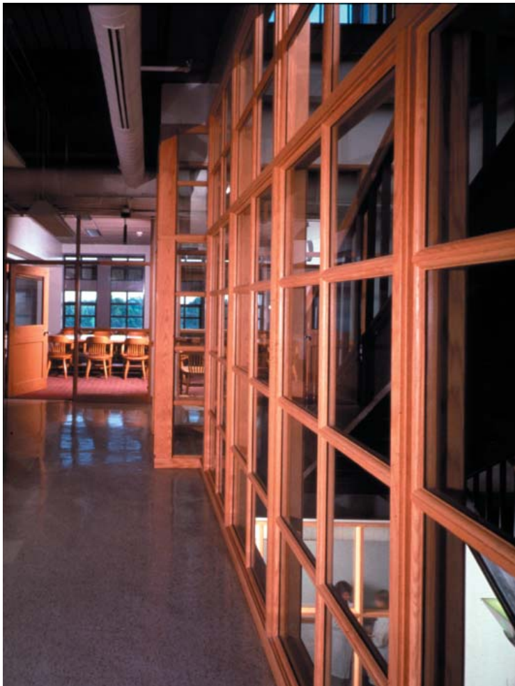
Central foyer and stairwell on the first floor of the Lewis Thomas Laboratory for Molecular Biology at Princeton University. The extensive use of glass brings "borrowed light" well into the building's interior. Here, light from the foyer and the distant conference room is brought into the enclosed stairwell, encouraging passers-by to stop and converse on the lower landing.
