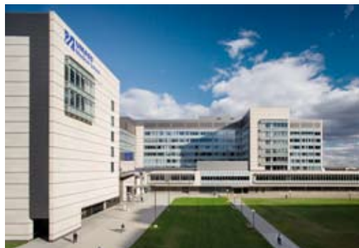
View of facade after Replacement
