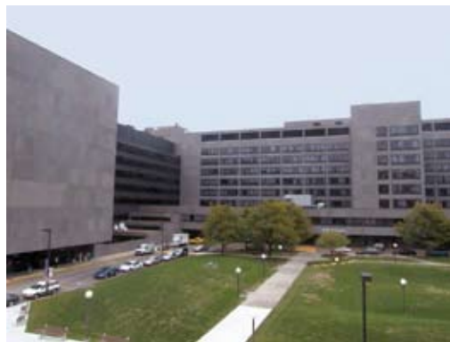
View of facade before Replacement
