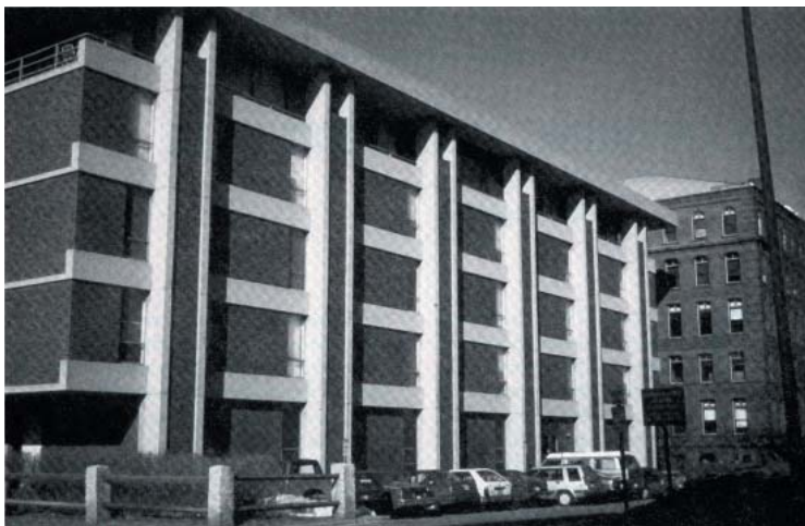
Many institutions constructed science buildings during the Sputnik era. The Hoffman Building at Harvard University is a typical example in its layout, materials, and systems.
